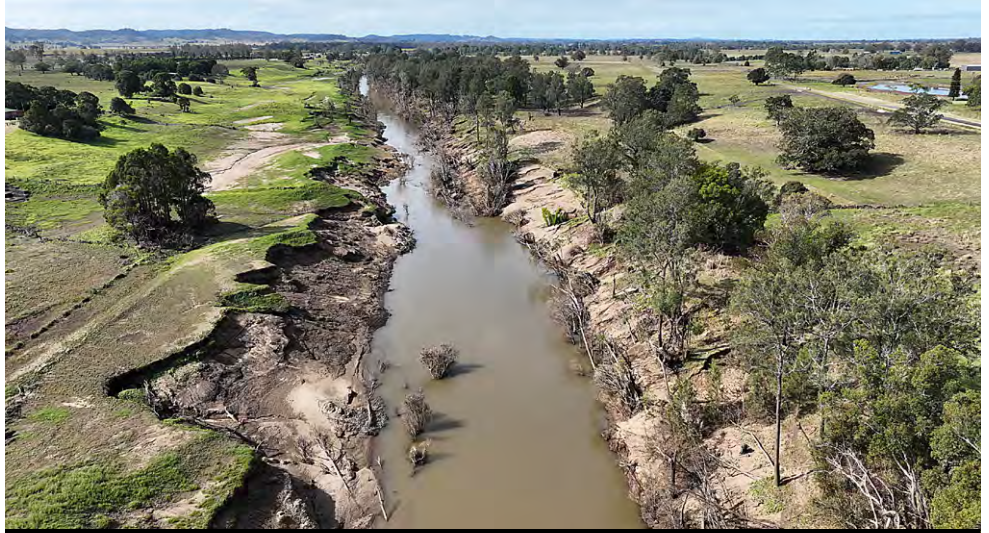
The Casino to The Channon river system showing signs of flood damage.
